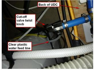
Rotate the cut-off valve arm 90 degrees away from the outlet of the valve to shut it off. Leave it that way until ready to use the icemaker again.
