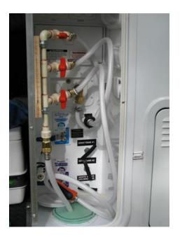
Here's an example of a simple manifold (shout out to JohnDar). Each output has a separate cutoff valve. There's a single input at the bottom of the manifold.
